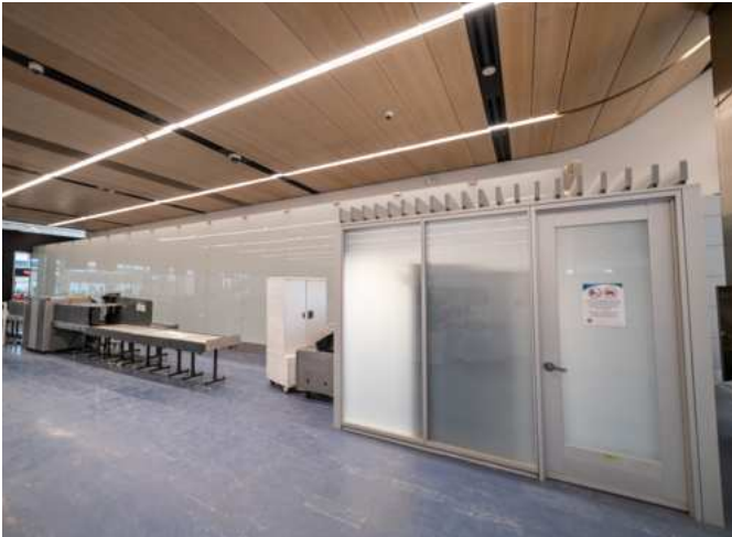
Check-In Walls: Designed 18-foot-tall freestanding walls with 1-inch thick glass.
