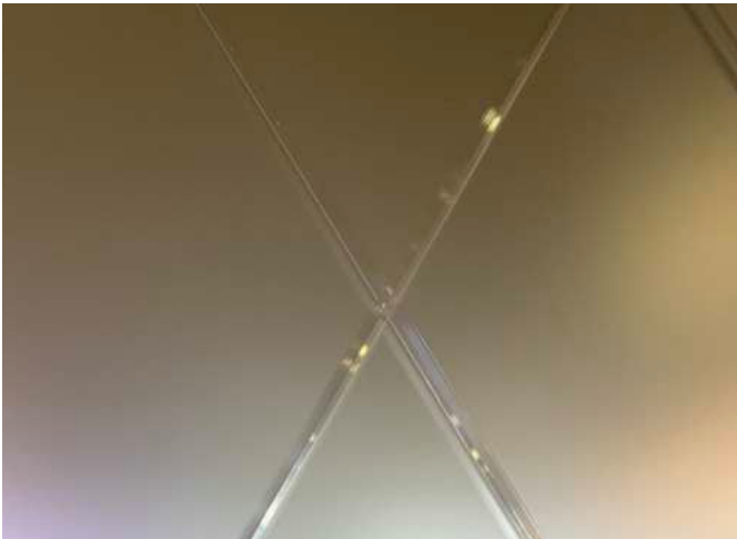
Custom Laminated Glass Panels: Installed with diamond pattern V-grooving for enhanced visual appeal.
