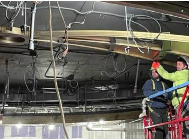
Lightweight Structural Support System: Engineered lightweight supports for dome installations at significant heights.
