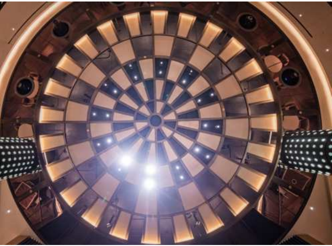
Prefabricated Dome System: constructed from aluminum with a metal plating finish, providing a lightweight yet visually impactful structure.
