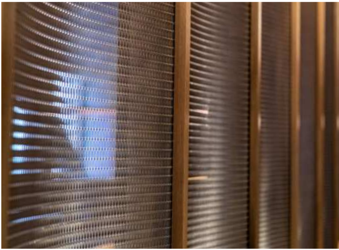
Custom Bronze Mesh Panels: Applied in doors and walls for aesthetics.
