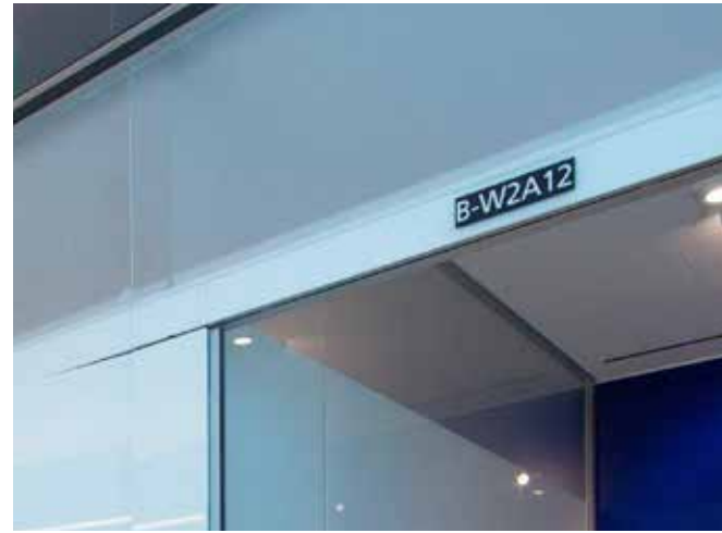
Custom Laminated Opaque Glass: Used for divider walls, featuring frosted tops.
