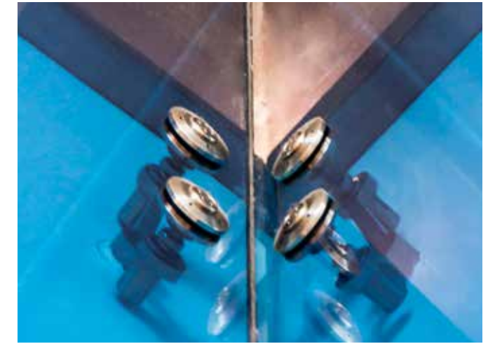
Stainless Steel Wraps: Mitered bars attached with double-faced tape.
