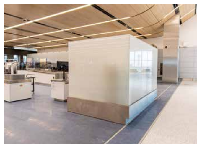
Security Modules: Utilized prefabricated stainless steel and glass modules for security kiosks and custom structural steel plates for security walls.
