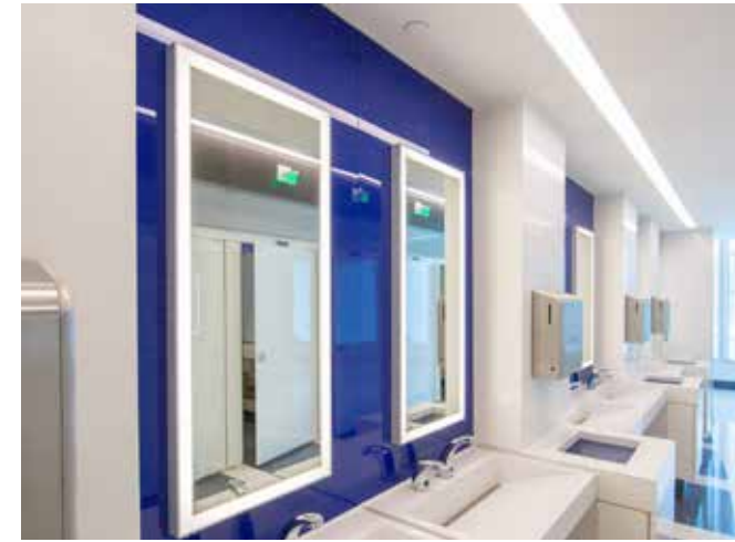
Back-Painted Glass: Installed at sinks behind back-lit mirrors.
