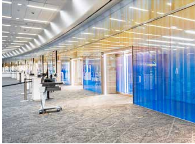
Structural Glass System: Utilized custom-fabricated laminated glass panels with precise curvature.
